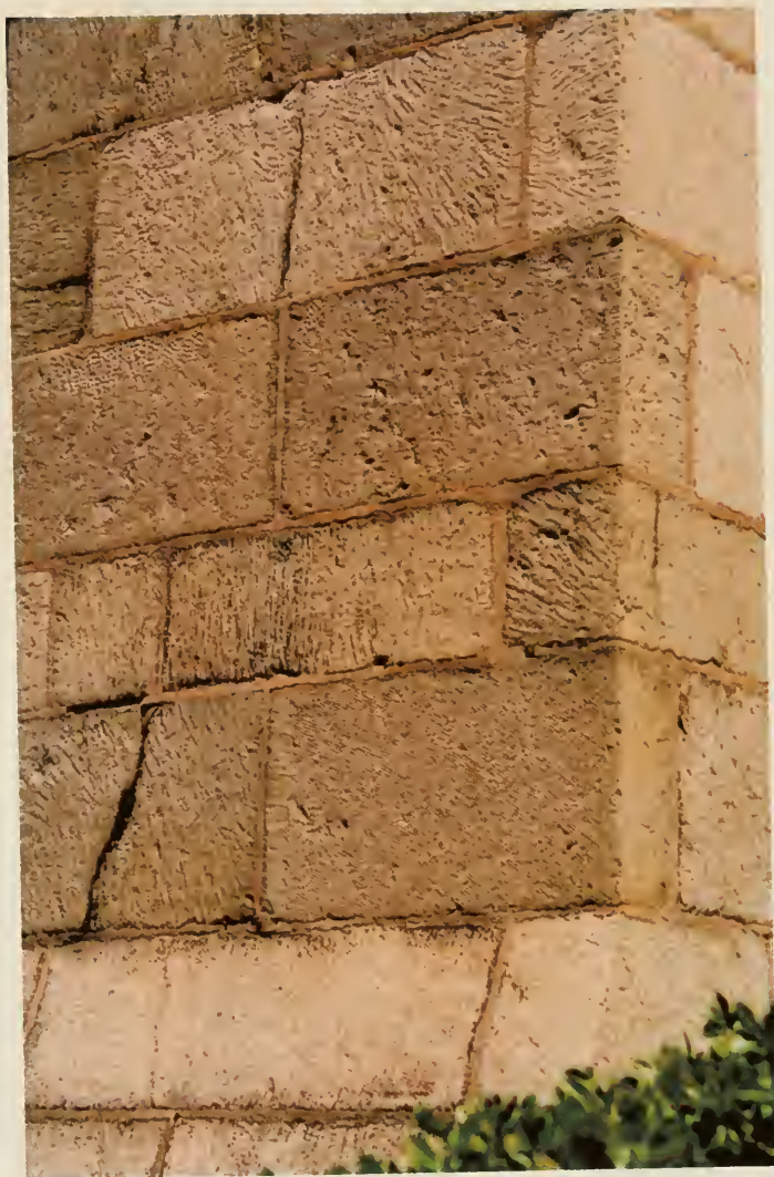
Photograph #36: Close-up of Horticultural Hall showing the blue coloring of its serpentine. Unfortunately, when exposed to direct and continual sunlight (the Hall faces west), blue serpentine tends to fade to a buff-green color. However, in certain kinds of lighting, such as indirect, the blue color can still be discerned.
